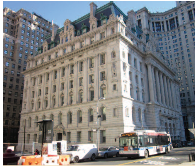
The New York City Public Administrator's Office, this year's Starnet Design Award "Unique Installation" category winner, was renovated throughout with low profile access flooring.
